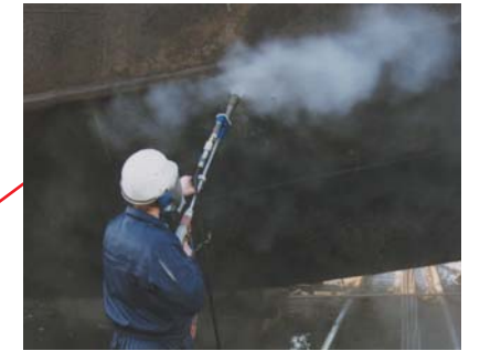
Weld seam cleaning and scale removal with the 3000-bar Modular Gun System.
