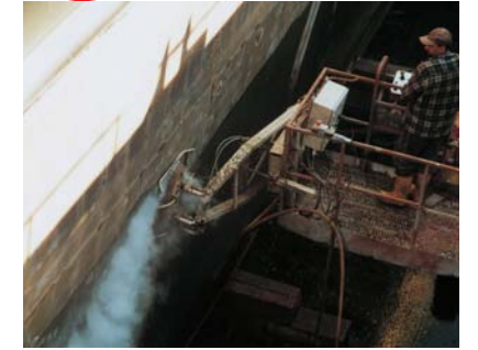
Emission-free mechanised large-scale surface preparation with the mechanical Triple Vacu Jet.
