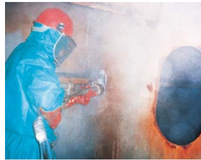
Ballast tank cleaning with the 3000-bar Modular Gun System.
