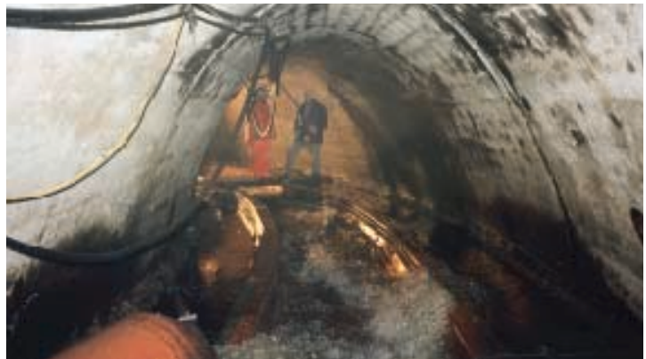
Removal of cement-based flat coat in man-sized channels by high-pressure water jet tools
