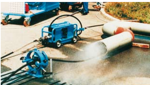
Internal pipe cleaning with TubeMaster®-System
