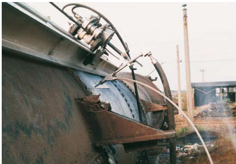
Vessel cutting with an abrasive ultra-high pressure water jet system
