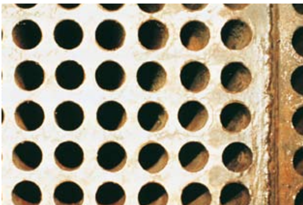
Heat exchanger cleaned by high-pressure water jetting
