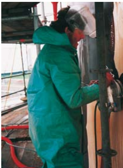
Emission-free paint stripping from tanks
